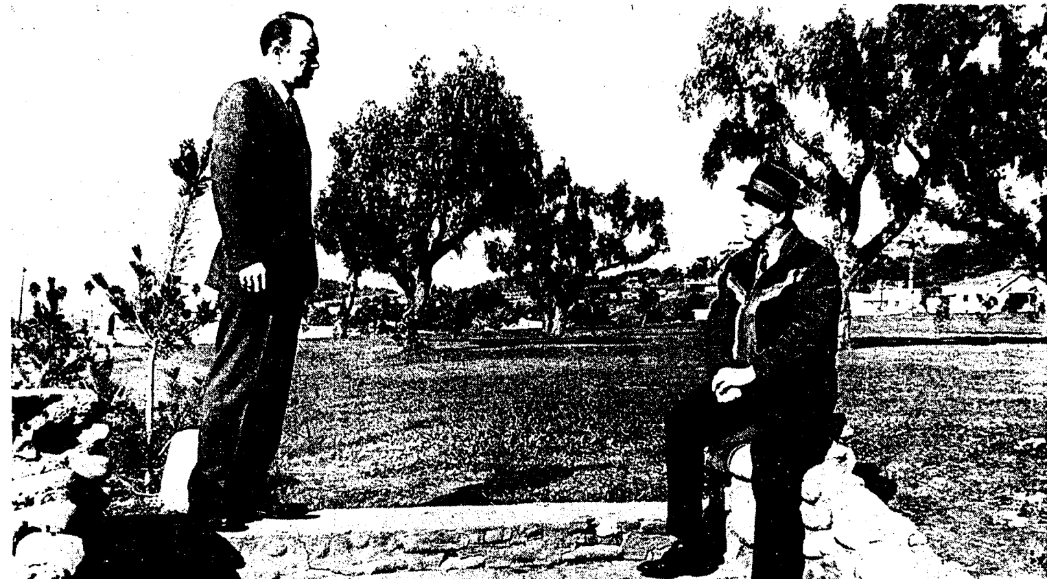
Former Ventura eyesore is now a spacious city park. In foreground, Bob Myers, left, city's administrative assistant, and Ed Lupton, park superintendent. Times photos by Kay Graham
